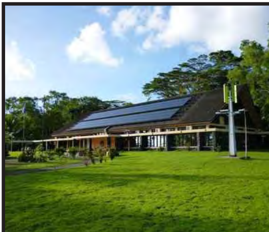
President's Office solar 70kW
