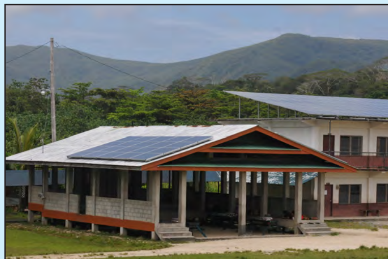
Nett Elementary School solar 200kW
