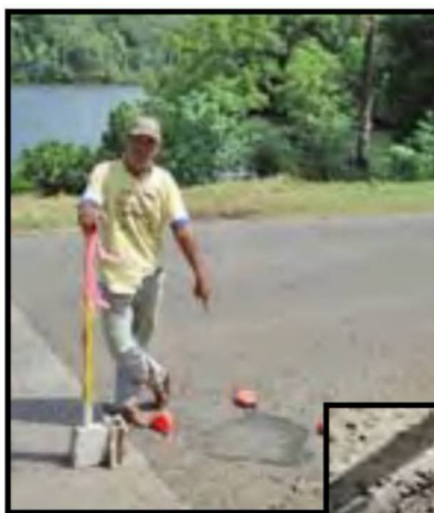
Repair near Dausokolo Bridge in Nett
