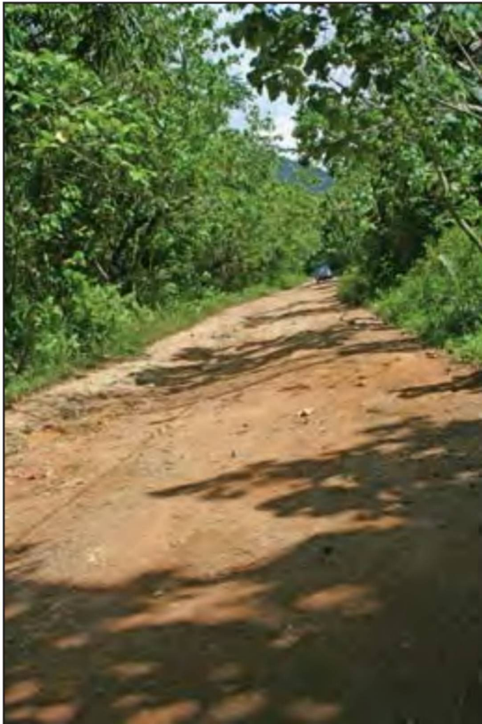
The unfinished Wone Elementary School Road
