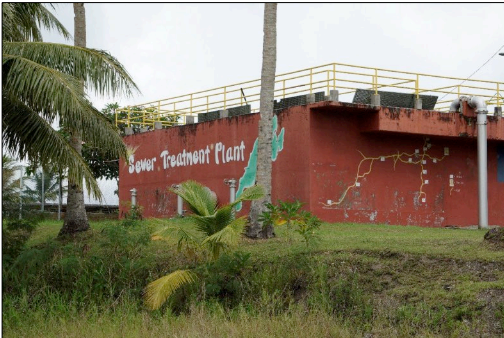
Photo 6. The sewer treatment plant in Yap Port Survey Area, facing east
