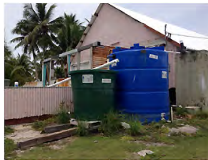
Water catchments and reversed osmosis units installed by IOM help the community salvage clean rainwater and transform salt water to drinking water.
