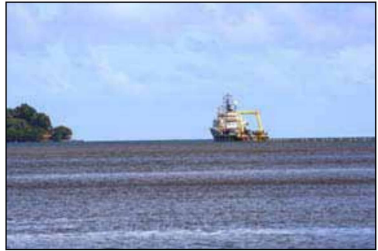
The Amarco Cheetah feeds cable while locally hired boats tow it. The cable is floated above the floor of the lagoon with inflatable buoys attached every 7 meters
