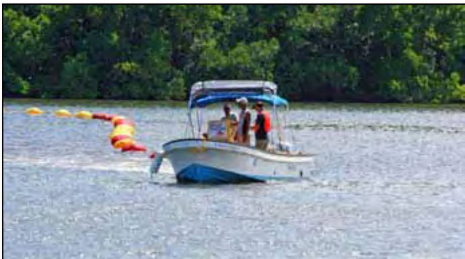
Locally hired boat tows the new fiber optic cable
