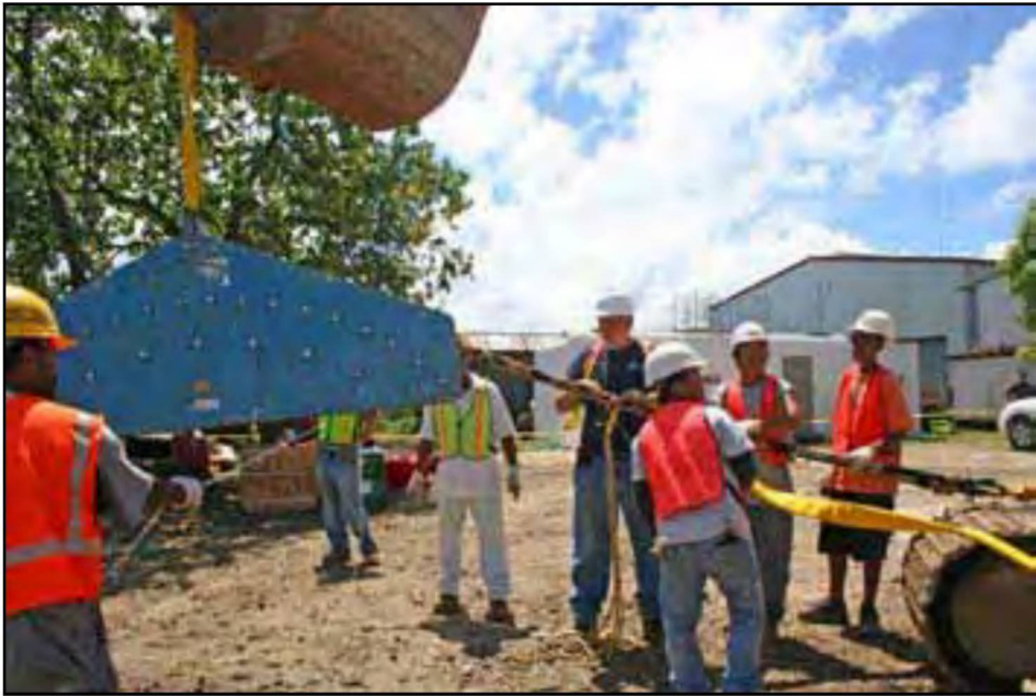
"Beach crew" works to secure the fiber optic cable on shore
