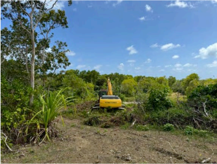
Photo 57. Active vegetation clearing east of airport.
