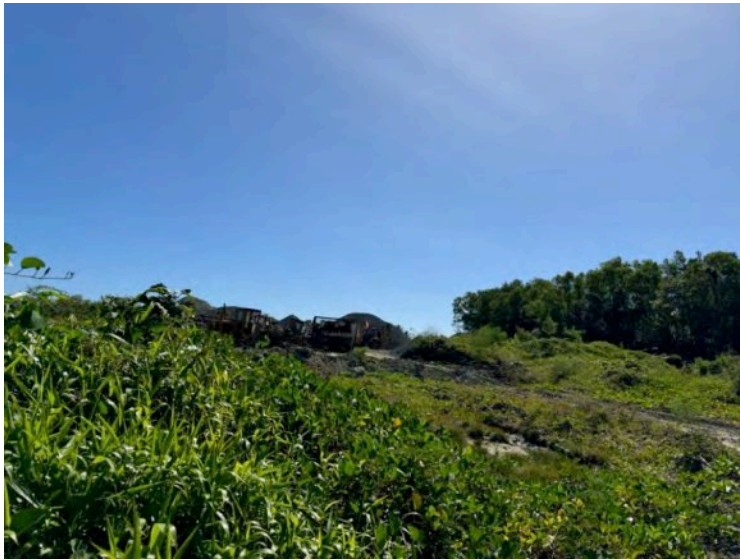
Photo 61. Construction area east of airport.
