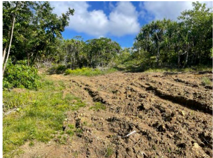
Photo 60. Cleared road east of airport.
