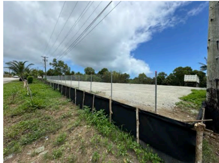
Photo 62. Construction staging area east of airport.
