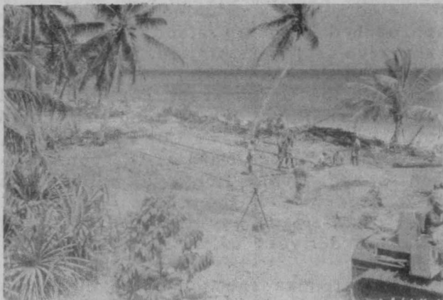
CONSTRUCTION - Forms being prepared for concrete floor slab of warehouse being built on Rongelap.
