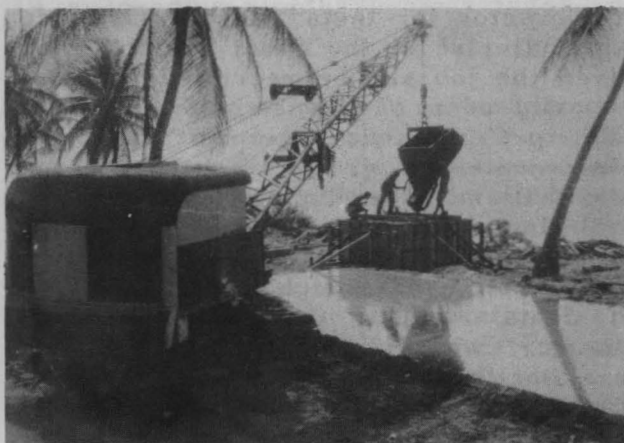
Construction Continuing - Pouring concrete in cistern.
