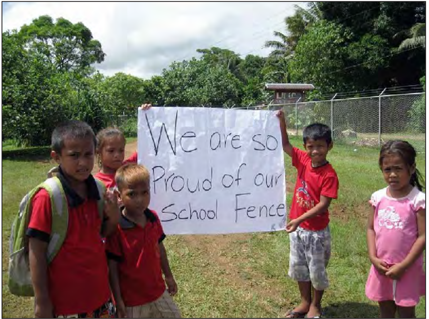
Lukop Elementary Students excitedly show visitors their new perimeter fence enclosing the school grounds, procured with an RD CF Program Grant
