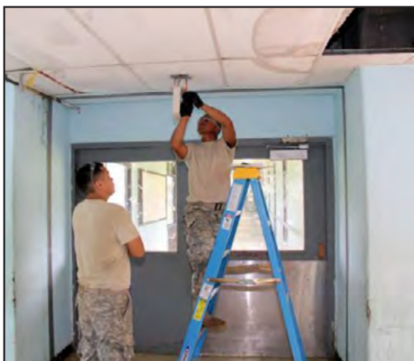
PFC Nedlic replacing an Exit sign
