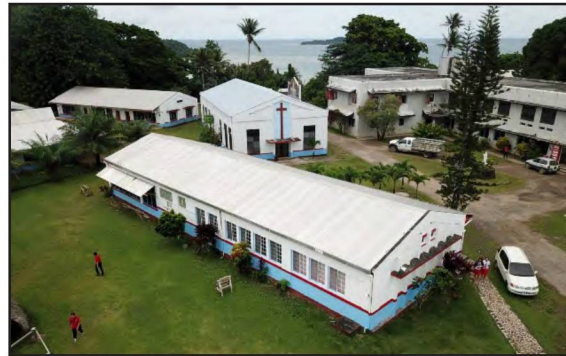
The Project for Reconstruction of School Library at Xavier high school in Chuuk State (Sep 2018)
