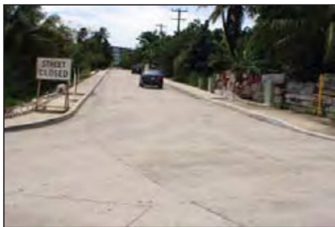
One section of completed road in Weno
