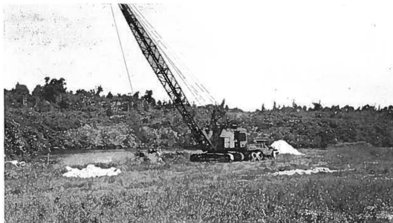
Drag-line excavator at West Lake. July, 1946.
