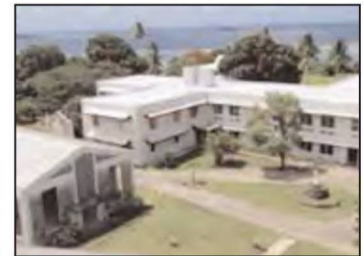
Xavier High School after renovation
