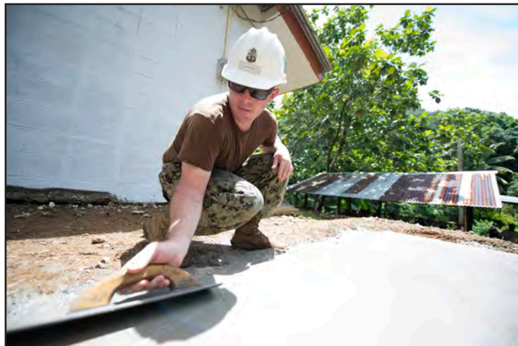
POHNPEI (June 25, 2015) – Chief Steelworker Bradley Vanhorn finishes concrete during a school renovation June 25. U.S. Navy photo by Mass Communication Specialist 1st Class Carla Burdt
