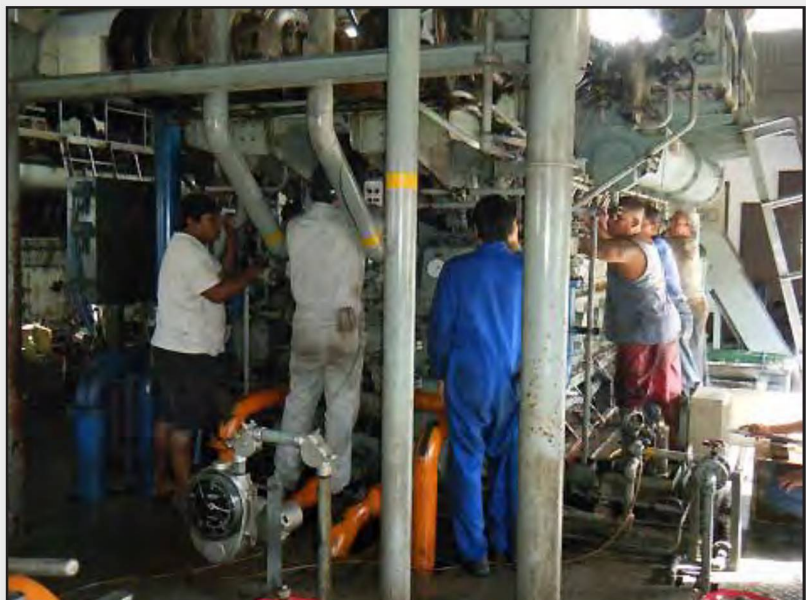
Contracted Japanese engineer, Ishizaki-san and Chinese engineer Xu Tao working together with the local PUC engineers on successful overhaul of No.9 generator.
