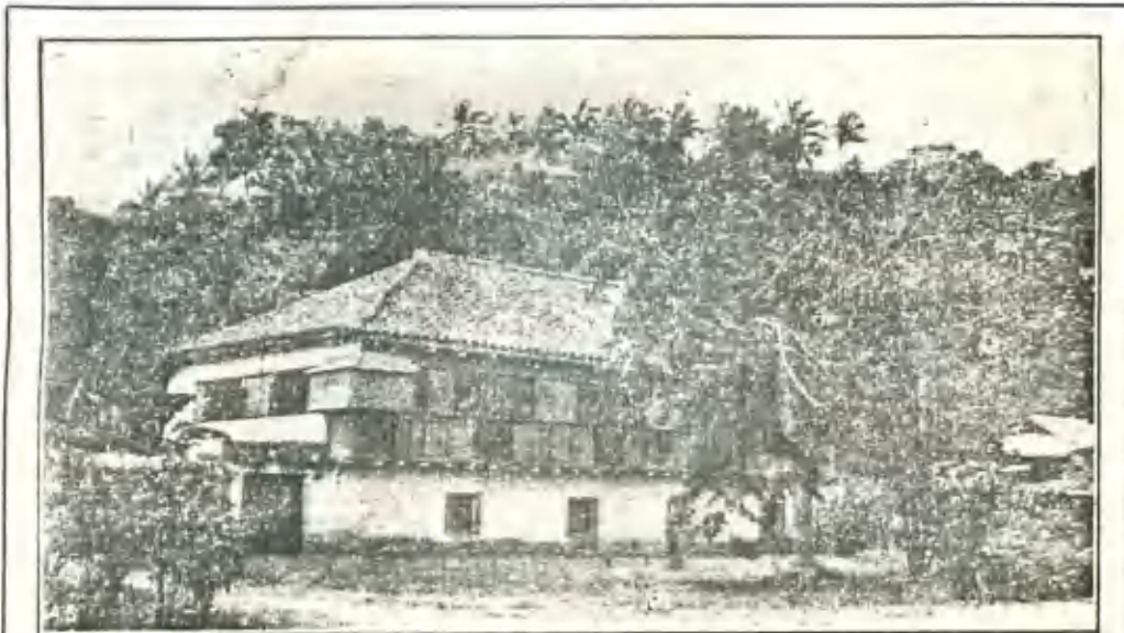
Spanish form of Architecture (Mamposteria, -lime and coral rock construction)
