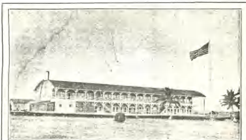
Photo by Mayhew U. S. Marine Corps Barracks, Sumay, Guam
