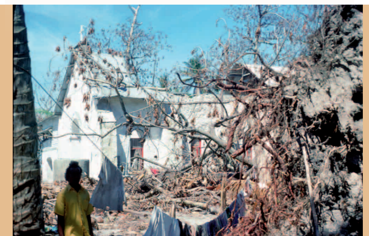
Kuttu church with typhoon damage in 1976
