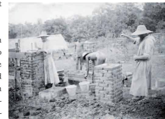
Br Ivo and another brother laying bricks for a new building on Pohnpei, c1910
