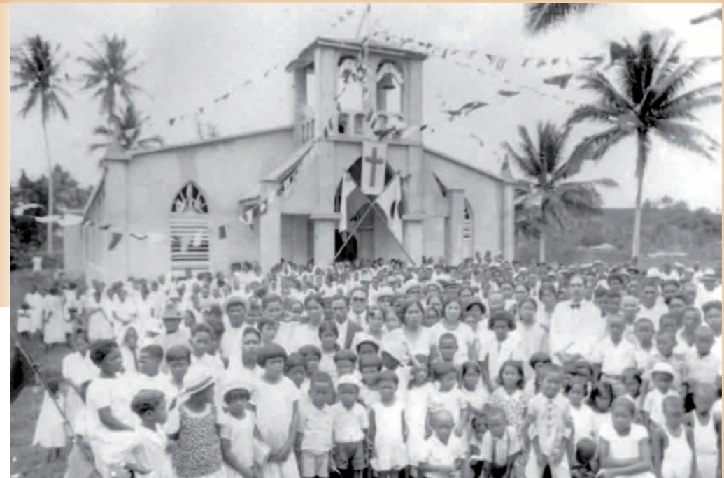
Dedication of the new Koror church in 1935
