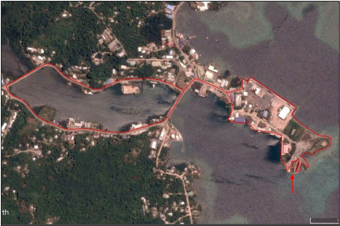
Photo 5: 2014 – Subject property, Colonia. The subject property looks generally the same from the last photo. The southeasternmost region of the subject property appears to be eroding. Red arrow points to region underwater.
