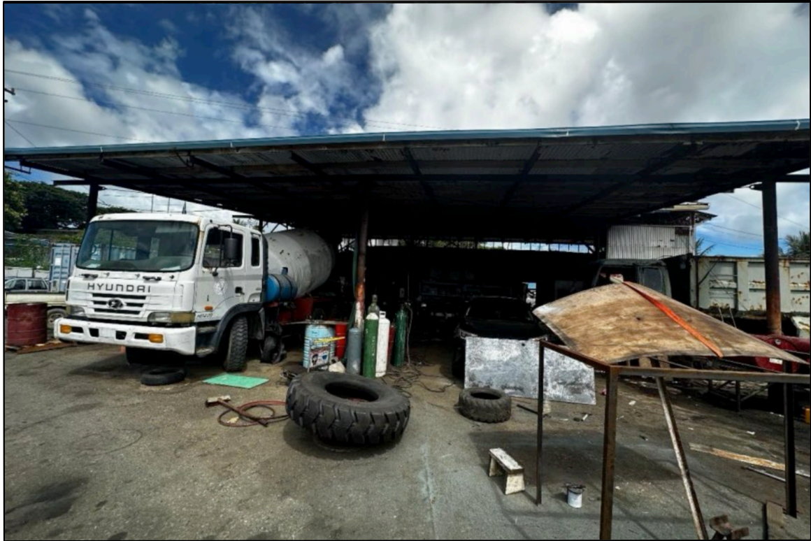
Photo 5: Overview of the Division of Sea Transportation maintenance shop. Photo is looking west.
