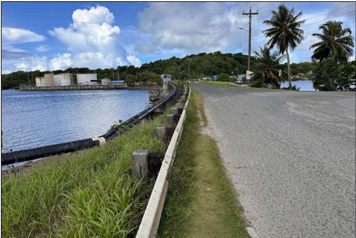
Photo 30: Small overpass leading to FSM Petroleum Corporation. Note: The subject property road is on the right and the fuel line is on the left. Photo is looking southwest.
