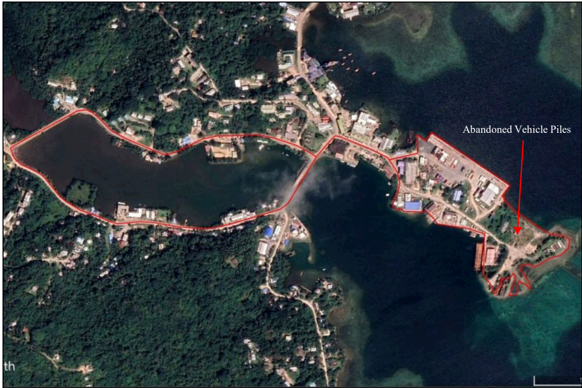
Photo 9: 2019 – Subject property, Colonia. The subject property looks generally the same from the last photo. The abandoned vehicle piles are beginning to accumulate (denoted by red arrow).
