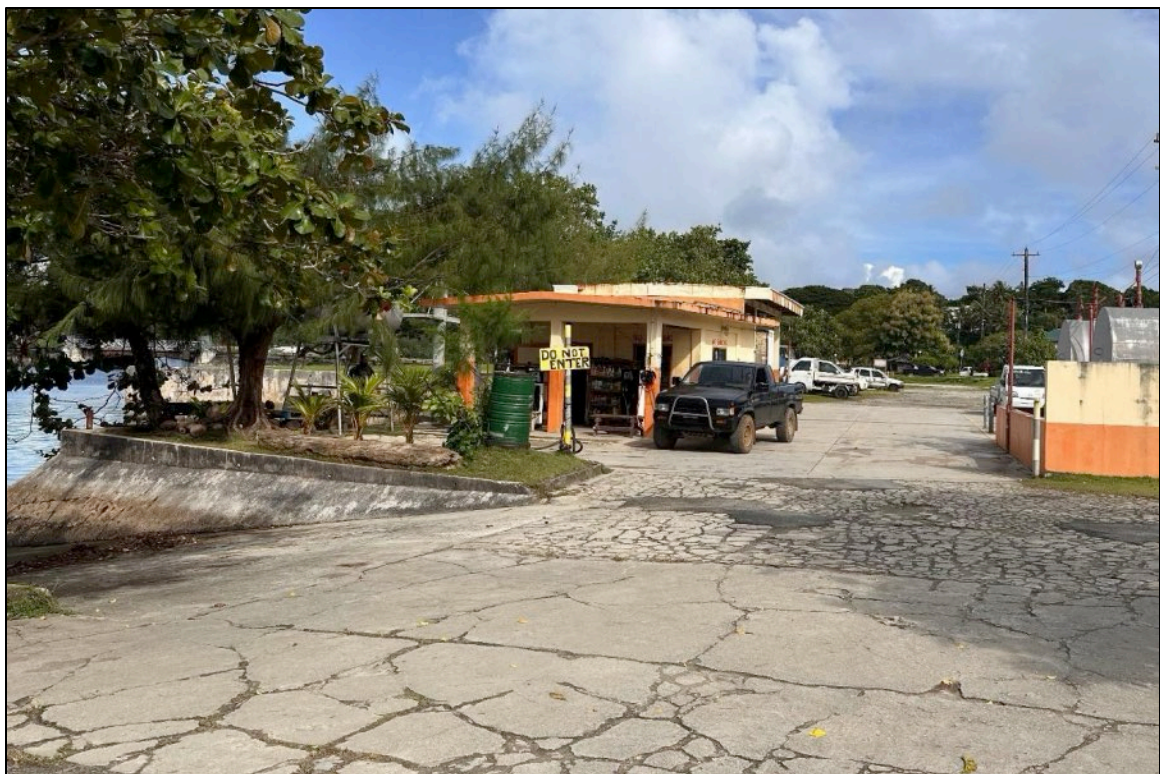
Photo 26: Overview of YCA Rufan Gas Station and its proximity to the ocean. Photo is looking southwest.
