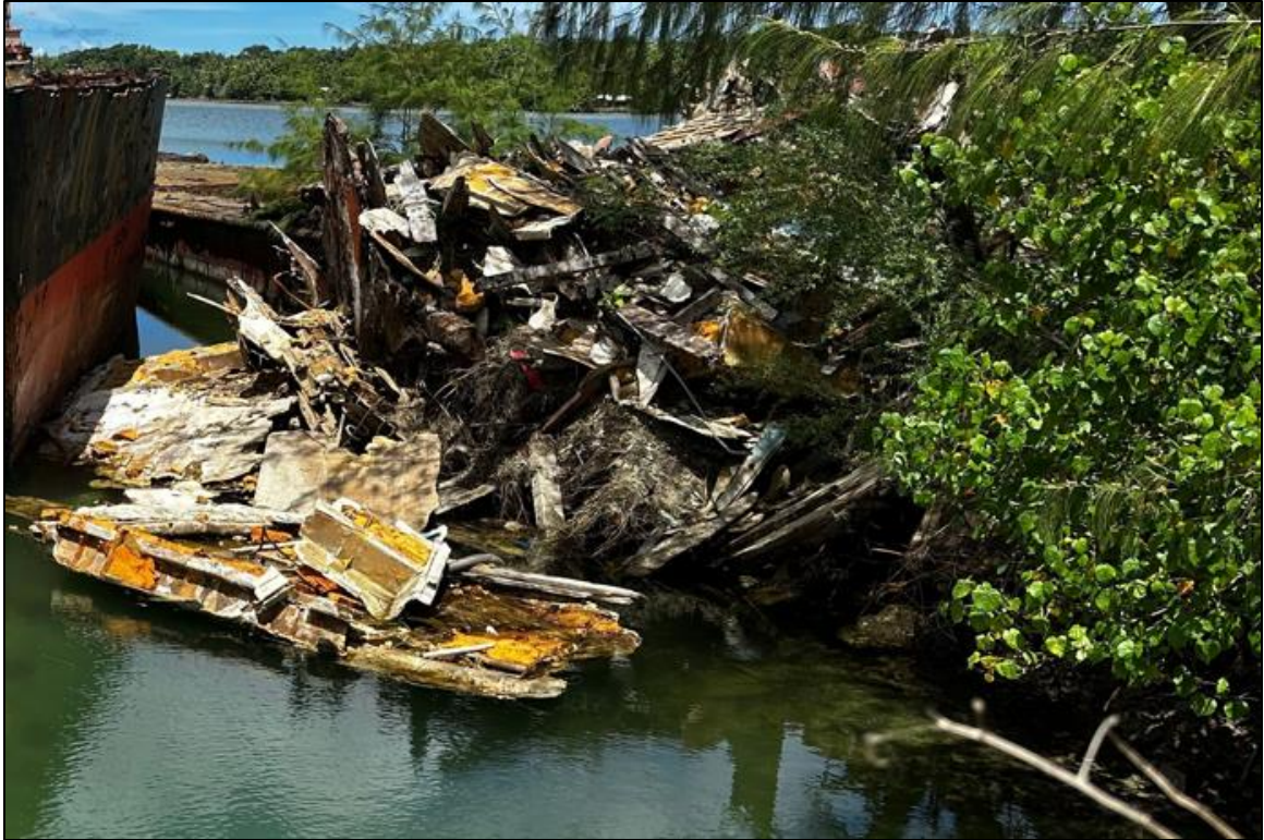
Photo 19: Overview of demolition debris mound located in the southeasternmost point of the subject property. A portion of the mound was observed eroding into the ocean. Photo is looking southeast.
