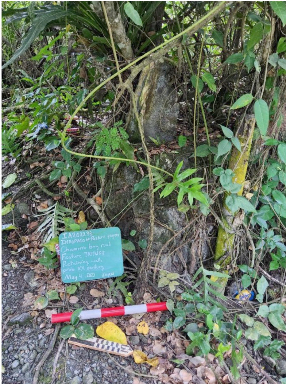
Figure 3-28 Temporary Site 02, Stone and Coral Retaining Wall in Woorwoo Village, Rull Municipality; View West
