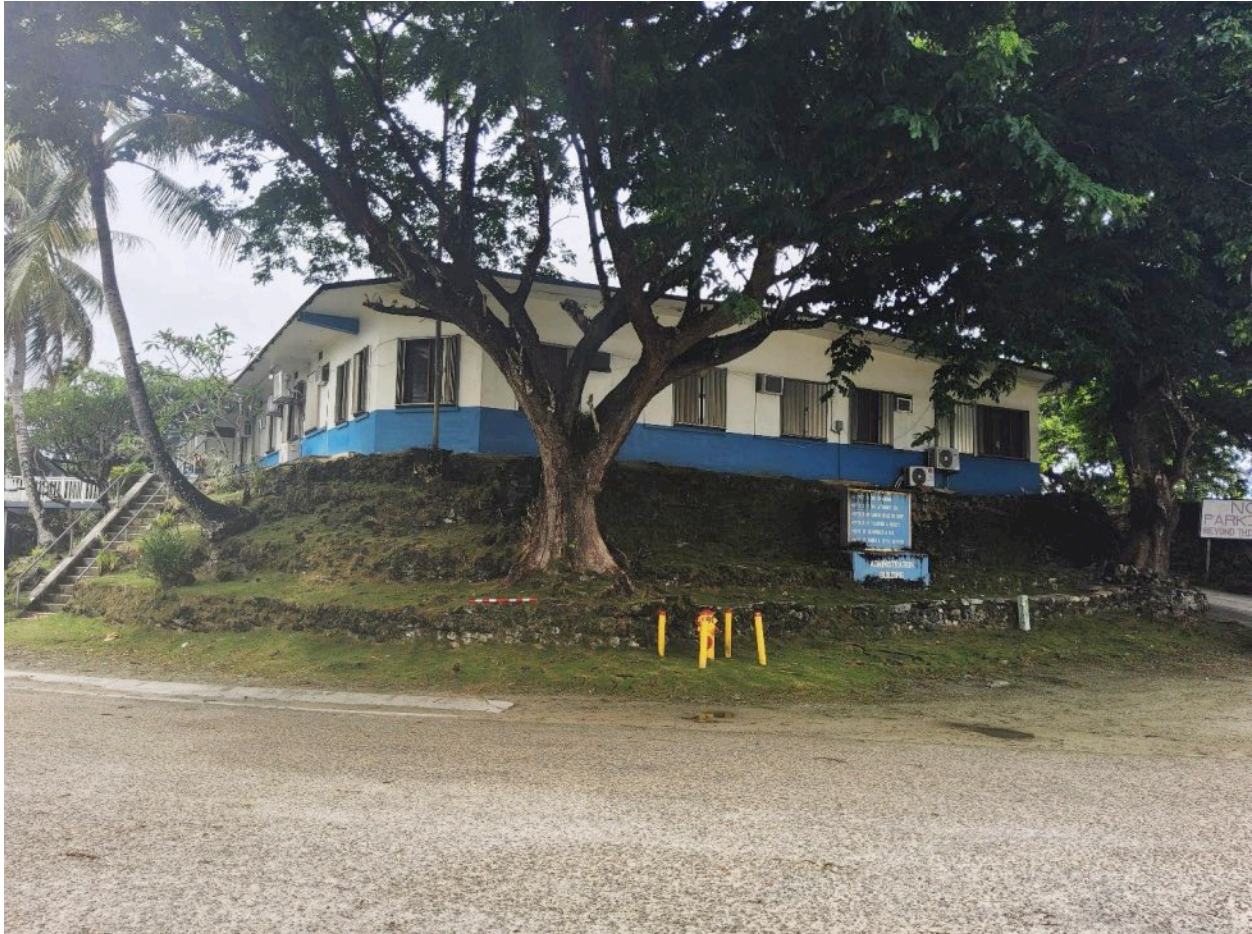
Figure 3-9 Feature 04, Traditionally Constructed Yapese Terraces Built along the South and West Sides of the Spanish Colonial Embankment and Mound (Feature 06); View Northeast; the Building is the Former Japanese Hospital
