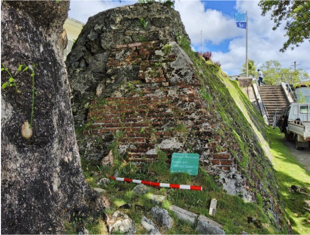
Figure 3-15 Feature 06, Southeast Corner Revealing Coursed Mortared Brick within an Interior Veneer and Cap of Mortared Masonry; View North
