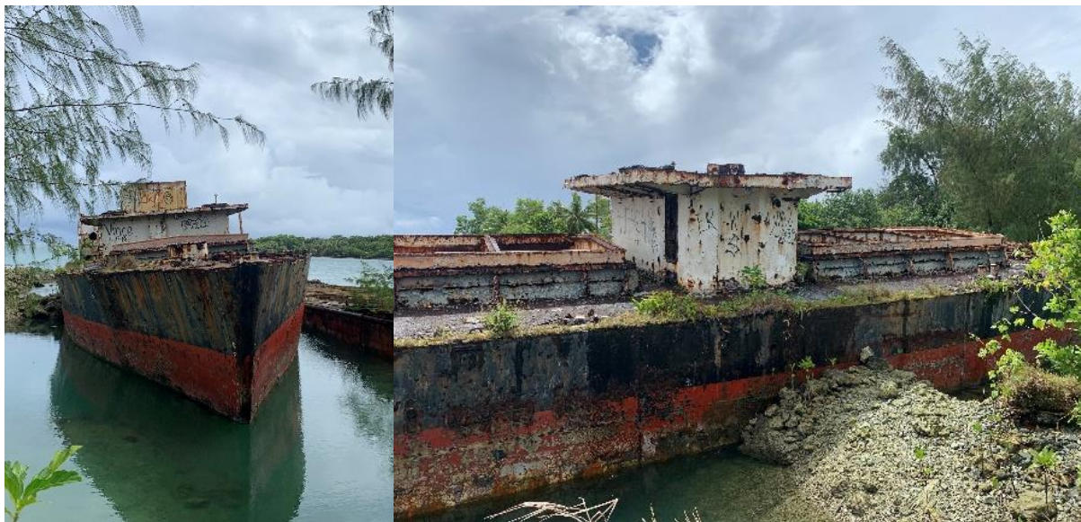
Figure 3-65 Weather Deck and Two Hatchways on Target 01 (Photo by AECOM)
