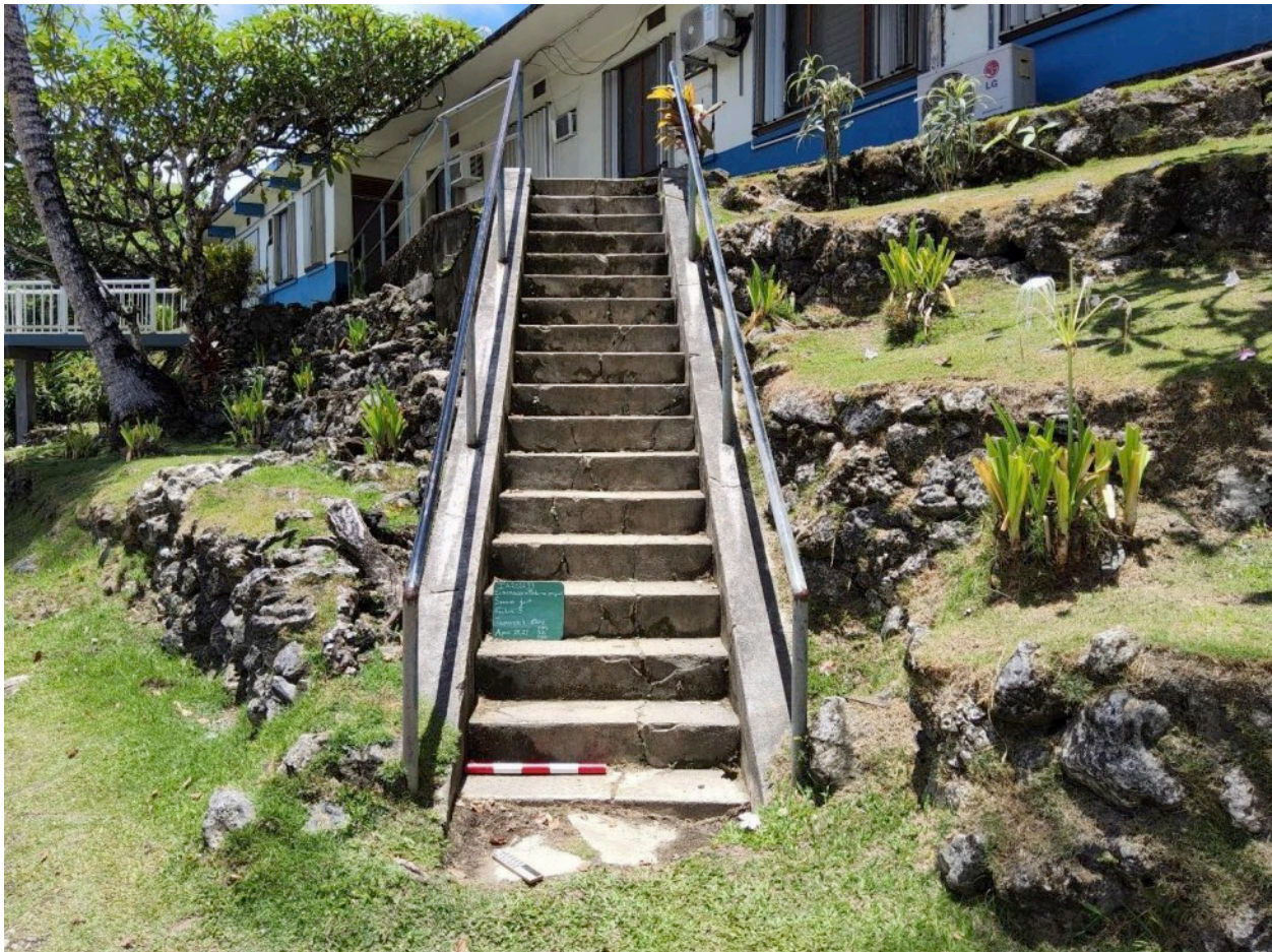
Figure 3-13 Feature 05, Japanese Staircase on the West Side of the Site; View Northeast
