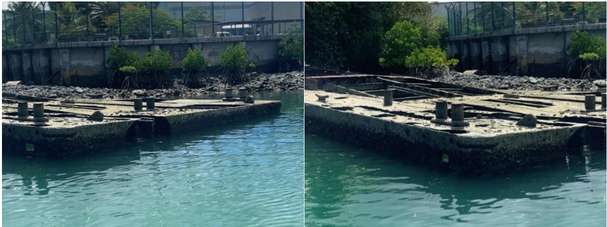
Figure 3-105 Target 15 (Photos by AECOM)
