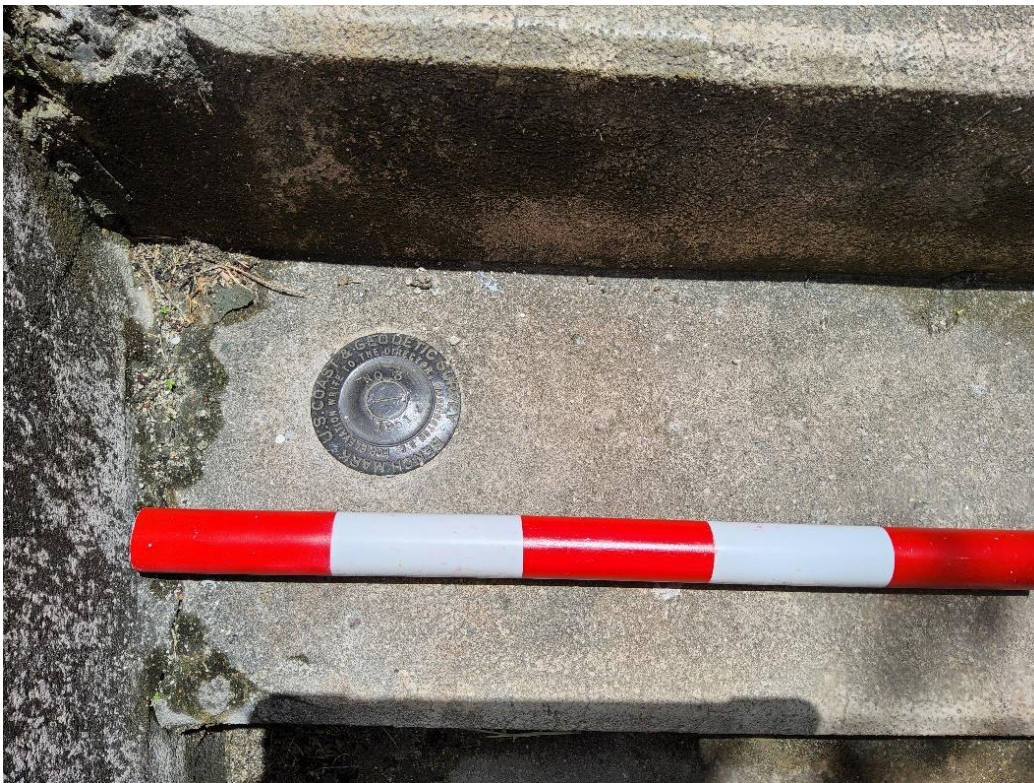
Figure 3-6 Feature 01, U.S. Coast and Geodetic Survey Benchmark, Installed in 1951, Embedded into One of the Steps of Feature 01
