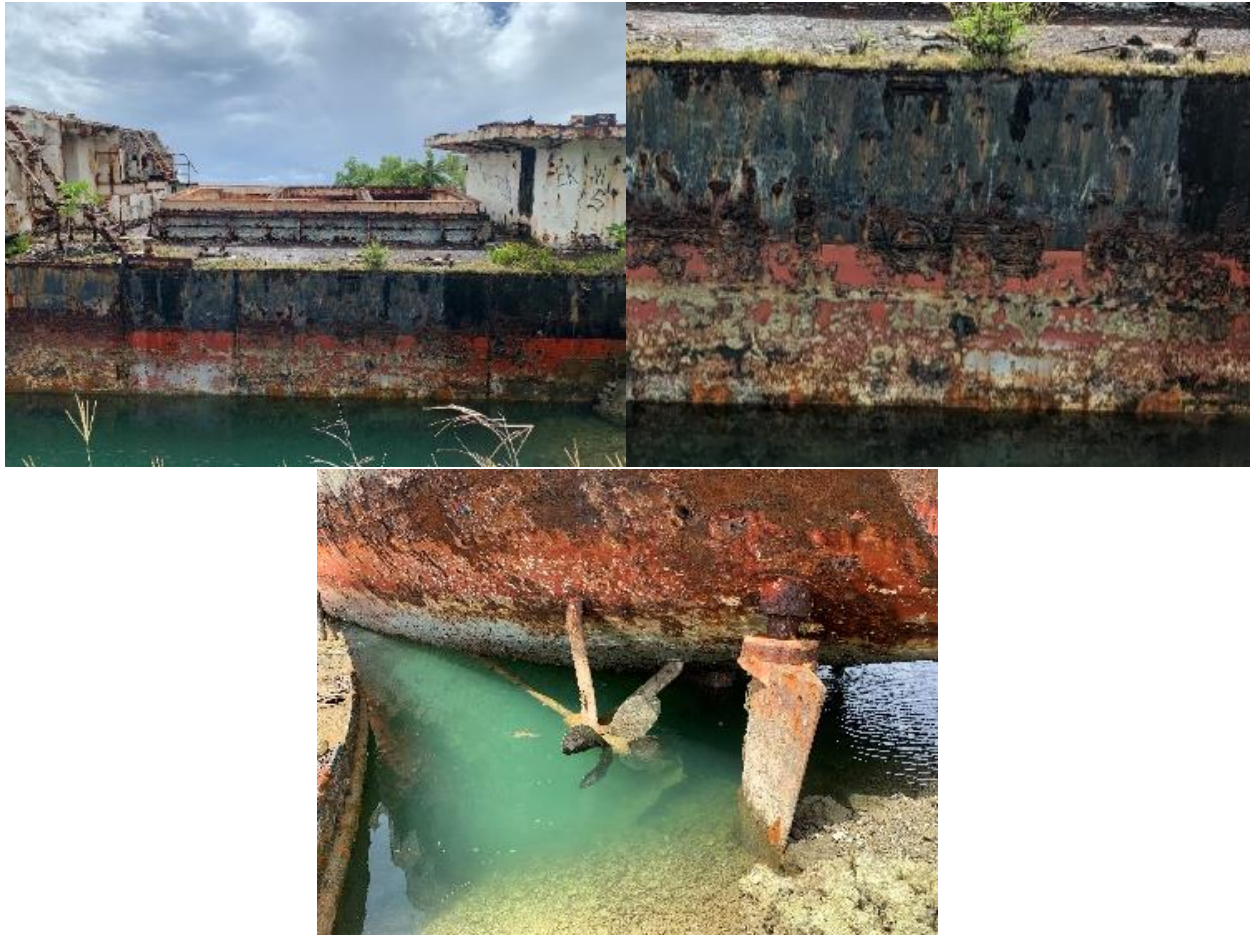
Figure 3-64 Welded Deck Plating, Plimsoll Mark, Fixed Skag, and Rudders on Target 01 (Photo by AECOM)
