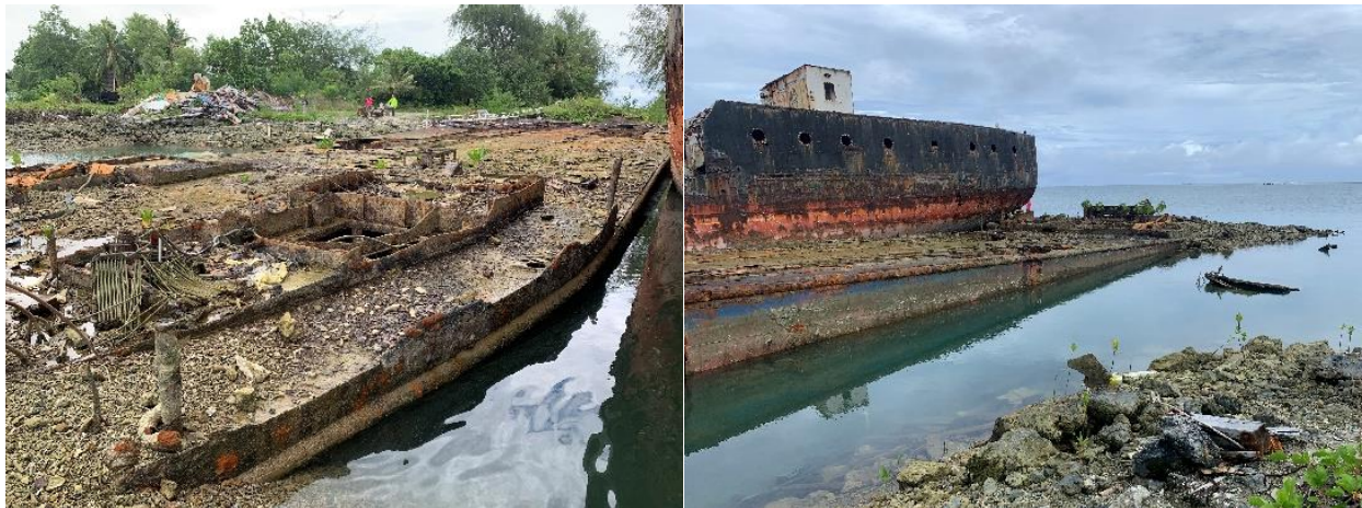
Figure 3-68 Target 02 (Photos by AECOM)
