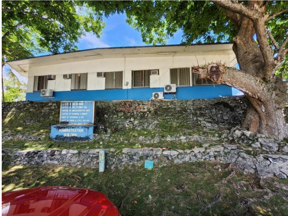
Figure 3-10 Feature 04, Traditionally Constructed Yapese Terrace Set along the South Side of Feature 06; View North
