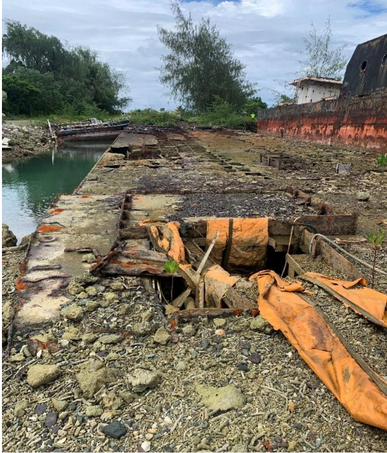
Figure 3-70 Evidence of Superstructure and Construction Elements of Target 02 (Photo by AECOM)
