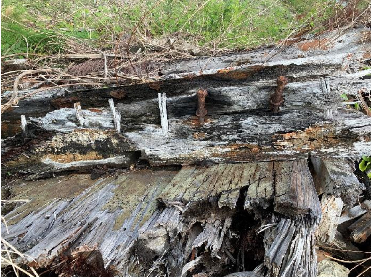
Figure 3-78 Treenails and Iron Bolts (Photo by AECOM)
