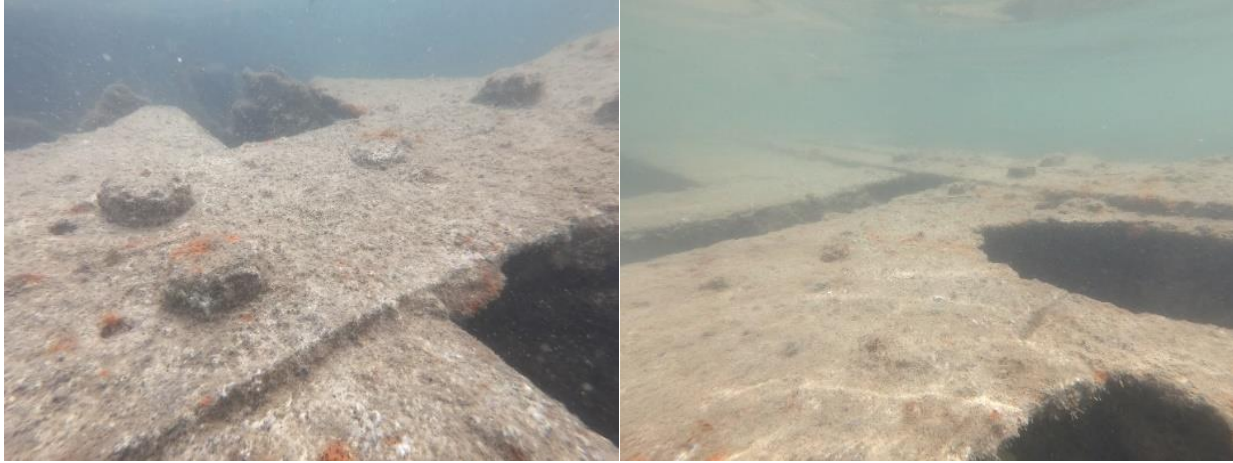
Figure 3-116 Single Riveting Butt Straps and Deck Plating (Photos by AECOM)
