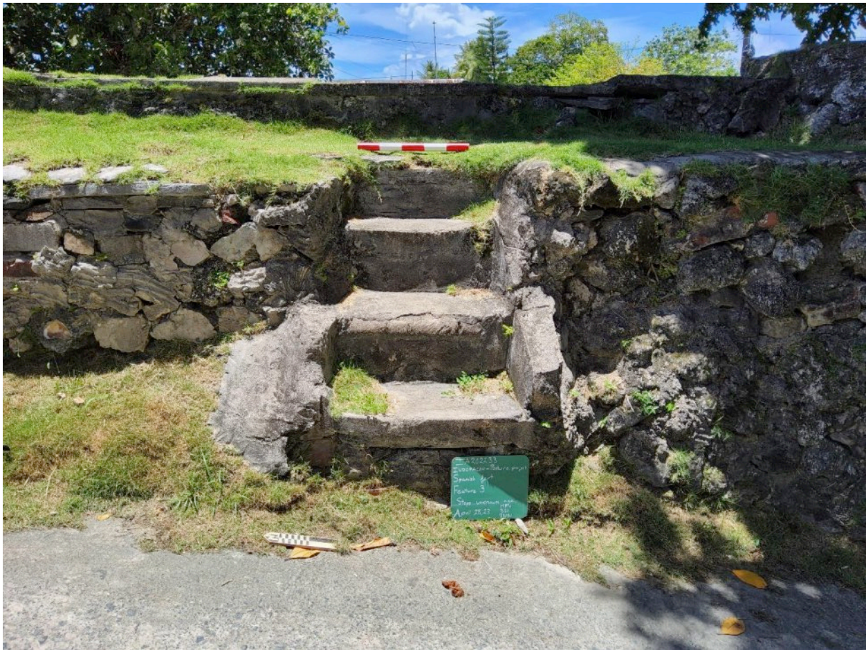
Figure 3-8 Feature 03, Sitting Area Comprised of Stairs, a Level Area, a Terraced Sitting Area, and Planters; View East
