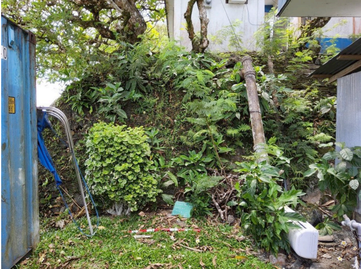
Figure 3-7 Feature 02, a Japanese Administration Drainage or Sewer Pipe at the Northwest Corner of the Site
