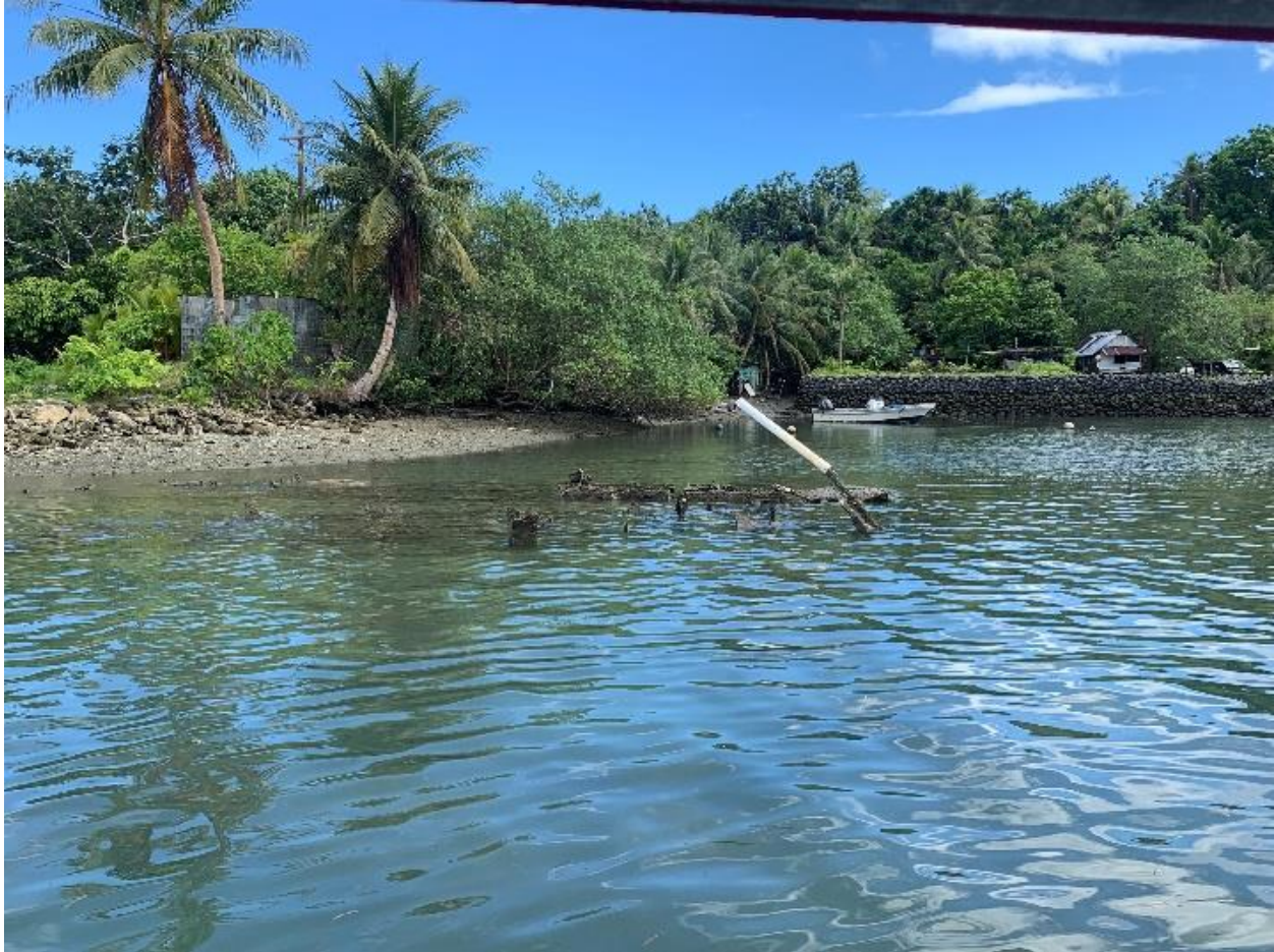
Figure 3-120 Framing Elements of Target 22 (Photo by AECOM)
