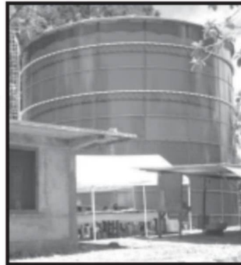
The 500,000 Gallon Tank in Kinakapw, Madolenihmw
